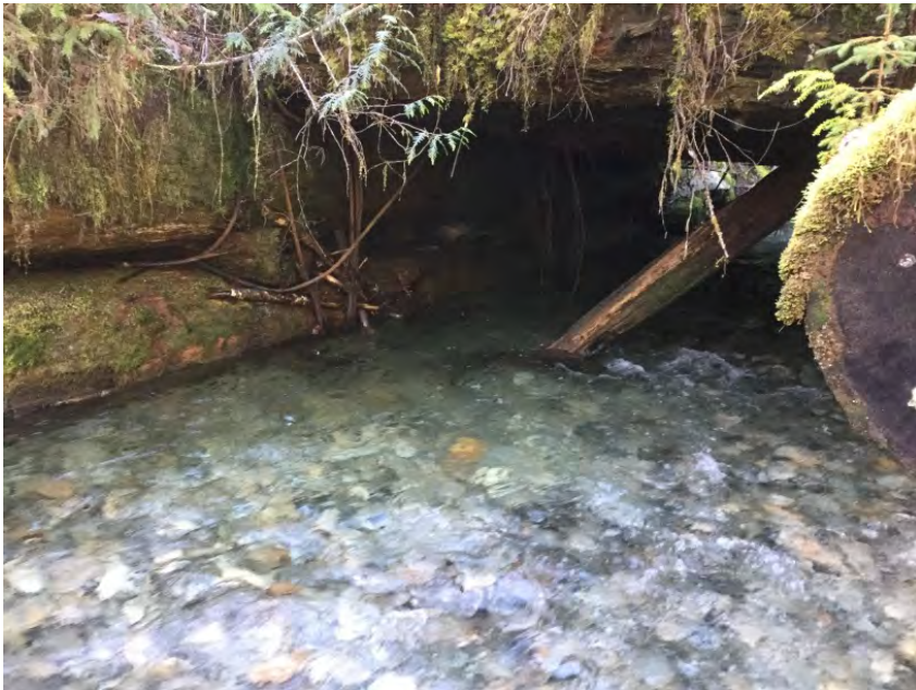
Right Bank Abutment when facing downstream
